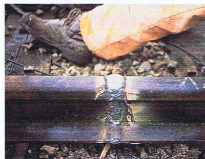
Fig.19 Complete weld before grinding
