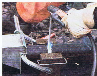
Fig. 18 Coppershoes mounted for mould welding of web and head
