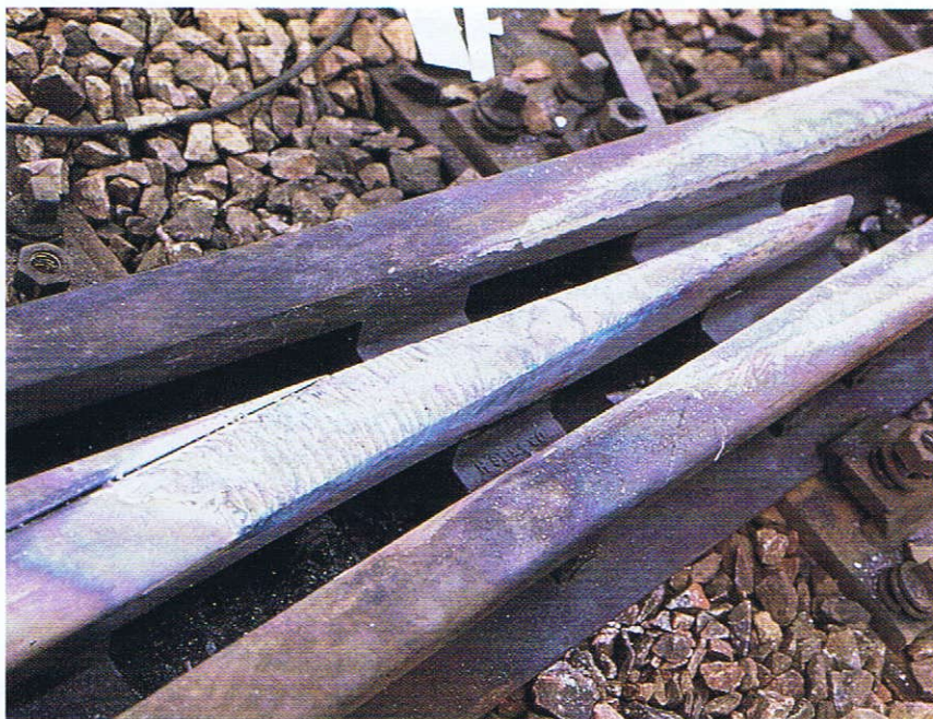
Fig. 23 Repaired C-Mn crossing before profiling
