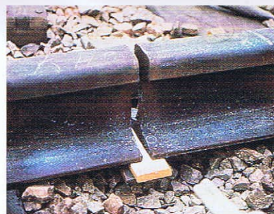
Fig.15 Mounting of backing.
